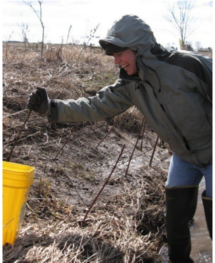
Live stakes should be positioned approximately 2-3 feet apart in several rows.
